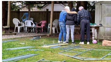
Installing greenhouse at Starr House.
